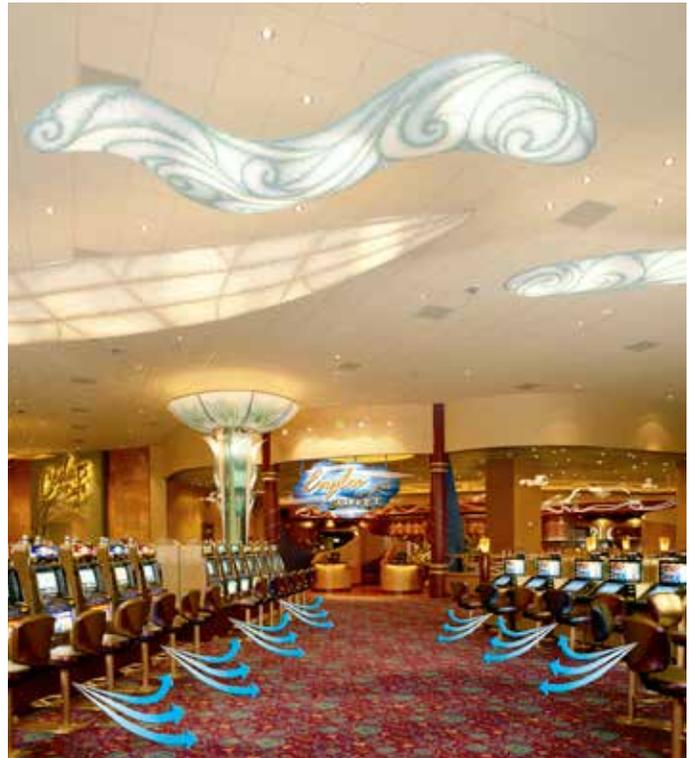
Underfloor Air Distribution with Air»Connect
